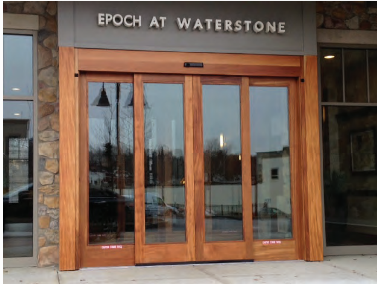
▶▶ 2000 Designer Package Epoch Senior Living & National Development. Mahogany wood doors and cladding. Architect: Elkus Manfredi | GC: Cranshaw Construction
